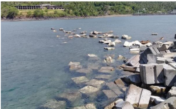
Concrete blocks scattered in the water
