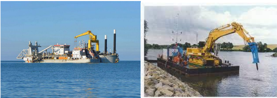
Figure 22 - Cutter + barge / BRH + barge
